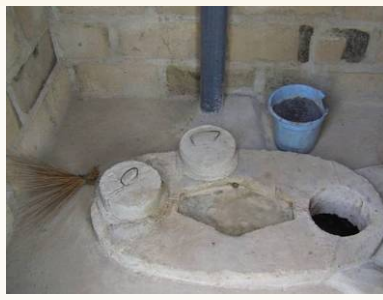
Urine separation integrated on the slab
