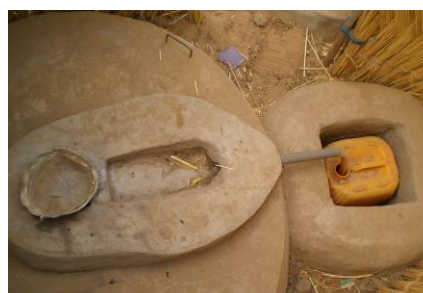
The composting toilet with urine diversion
