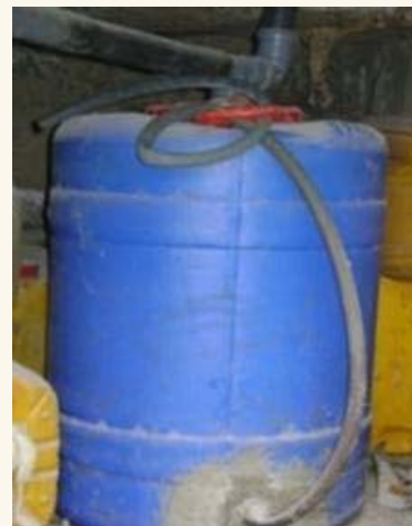
Figure 1: Typical storage tank in UDDT toilet
