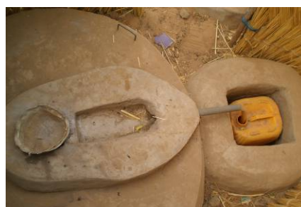
The composting toilet with urine diversion
