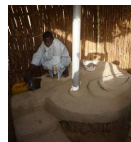
The dry toilet in local material except the slab and vent pipe.
