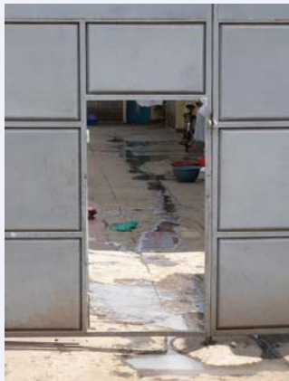
Figure 4: Greywater disposal in Nakuru
