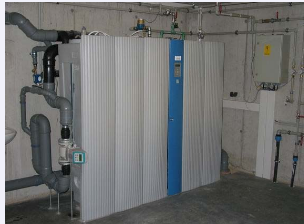
Figure 2: PONTOS Aquacycle 1500, SBR greywater treatment
