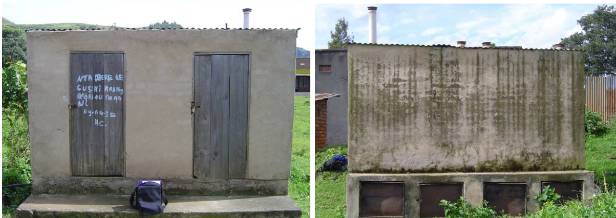
Figure 6.13.: Twin - double vault dry toilet. (f.l.t.r.) Front view. Rear view.
