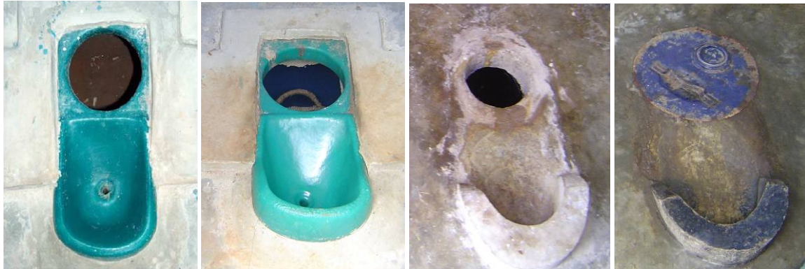
Figure 6.5.: Squatting pans. (f.l.t.r.) 1 st and 2 nd picture: Plastic pans in Kalungu. 3 rd picture: Concrete pan in kisoro. 4 th picture: Concrete pan with a lid in Kisoro.
