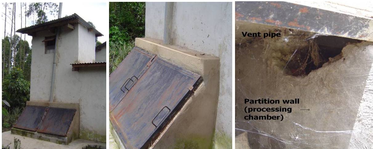
Figure 6.16.: (f.l.t.r.) Rear view (slanting doors; one outside vent pipe). Processing chamber doors. View inside the left Chamber with the bottom of the vent pipe as indicated.
