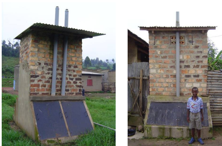
Figure 6.3.: Rear view of double vault dry toilets in Kabale. Left picture represents a double vault toilet with two vent pipes. Right image shows a double vault toilet with one vent pipe for both chambers.
